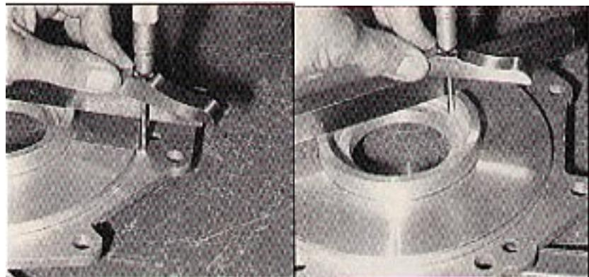
19. (above left) Lay the straightedge over the rear side of the front adapter plate. Use the depth micrometer to measure the distance from the top of the bar to the adapter plate mating surface and record the reading.
