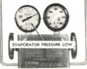
FIGURE 7—TXV STUCK CLOSED
