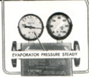
FIGURE 6—POA VALVE STUCK CLOSED
